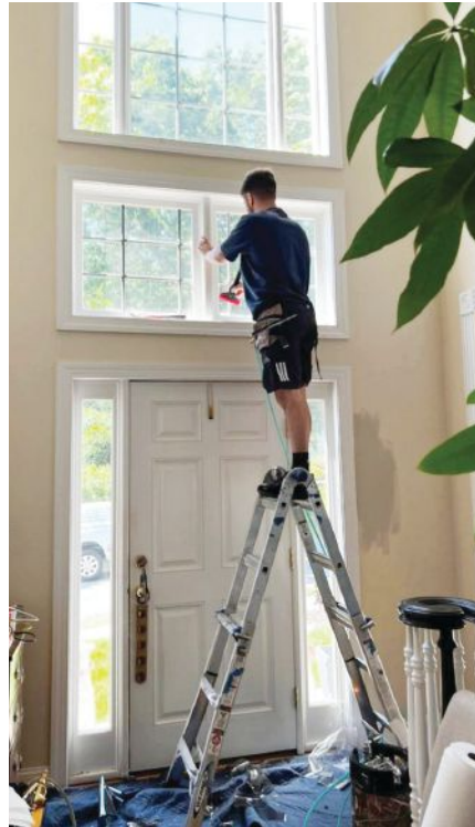
A member of Joe DelGiorno's team installs residential film.
